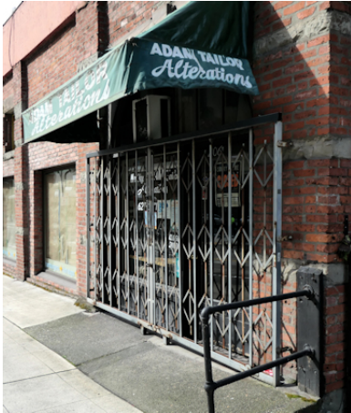
Figure xxx. Security bars and gates such as this detract from the area’s pedestrian qualities and are prohibited.
