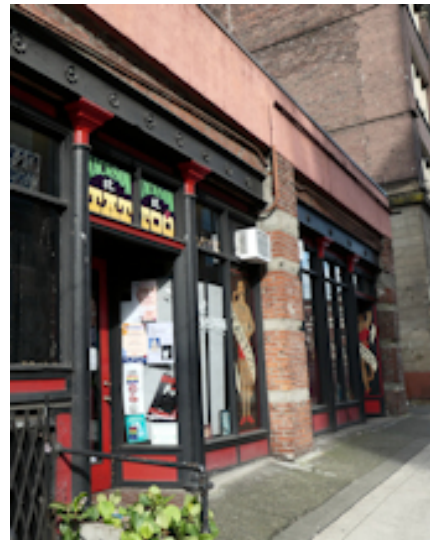
Figure xxx. Some buildings feature cast iron elements.
